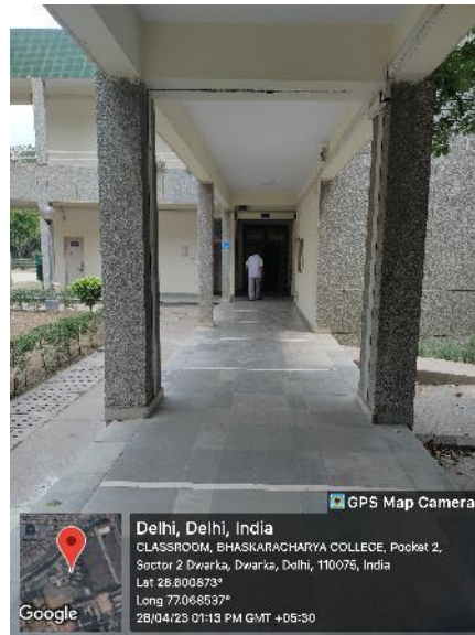
LED Panel Lights in Corridors
